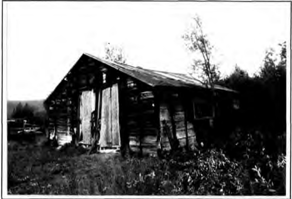
Figure 29. The Mutchler/Uotila/Fullerton Barn, 1993. The view is looking northwest.
